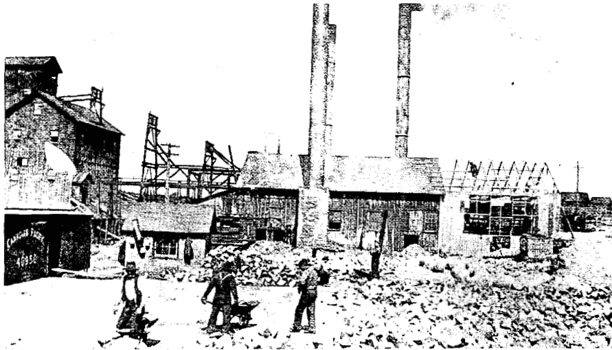
Canadian Copper Company, Copper Cliff. Matte yard, West Smelter as it was in 1902. The buildings were destroyed by fire June 14, 1904.
