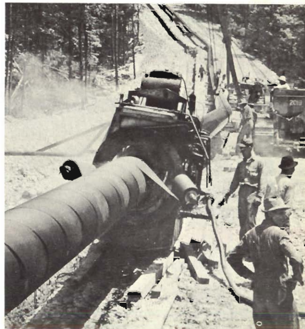
Pipelines carry gas and liquid fuels across the country to homes and factories. This pipeline will transport natural gas from Texas to West Virginia.
