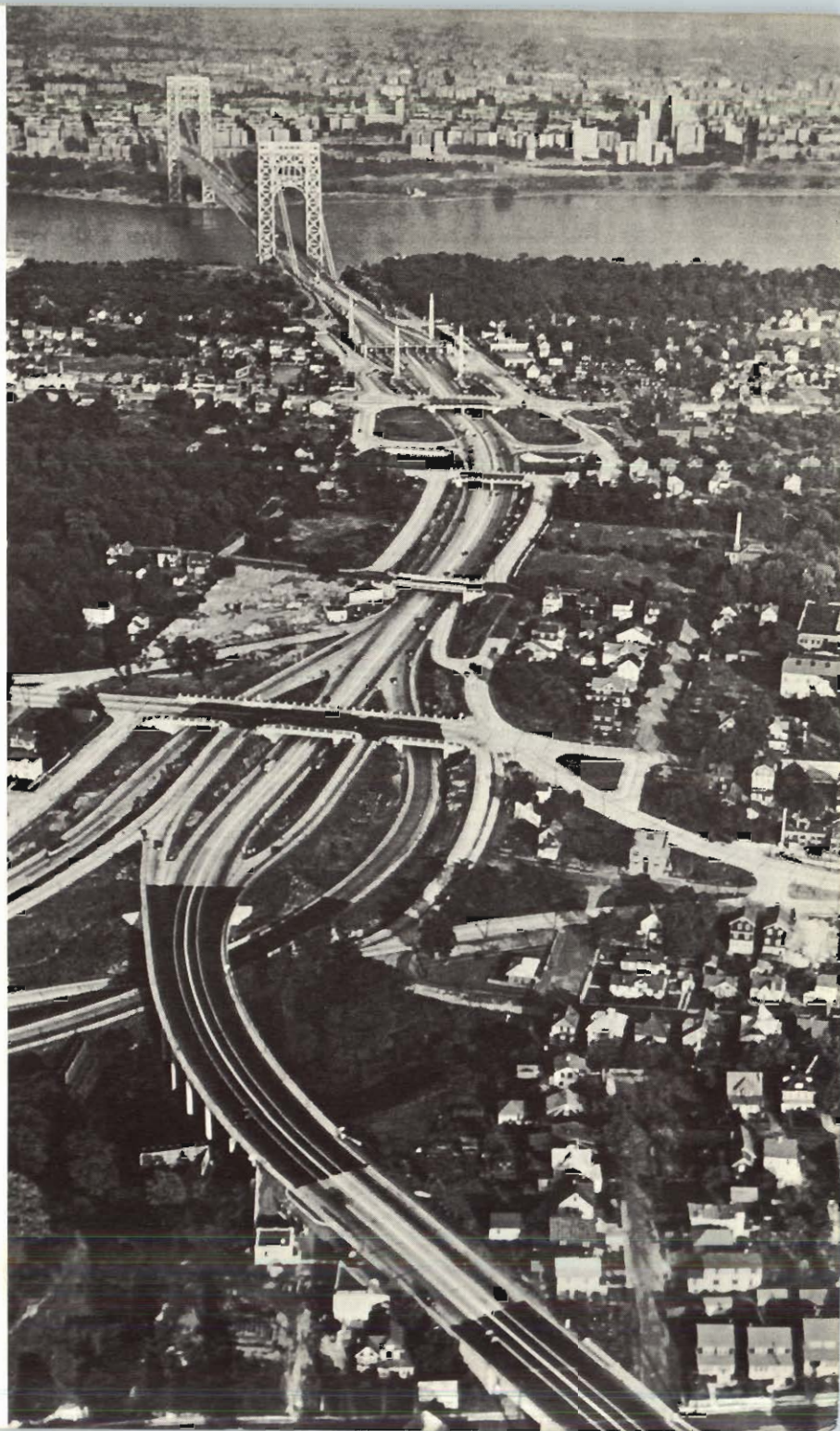
A highway network converges in New York City.
