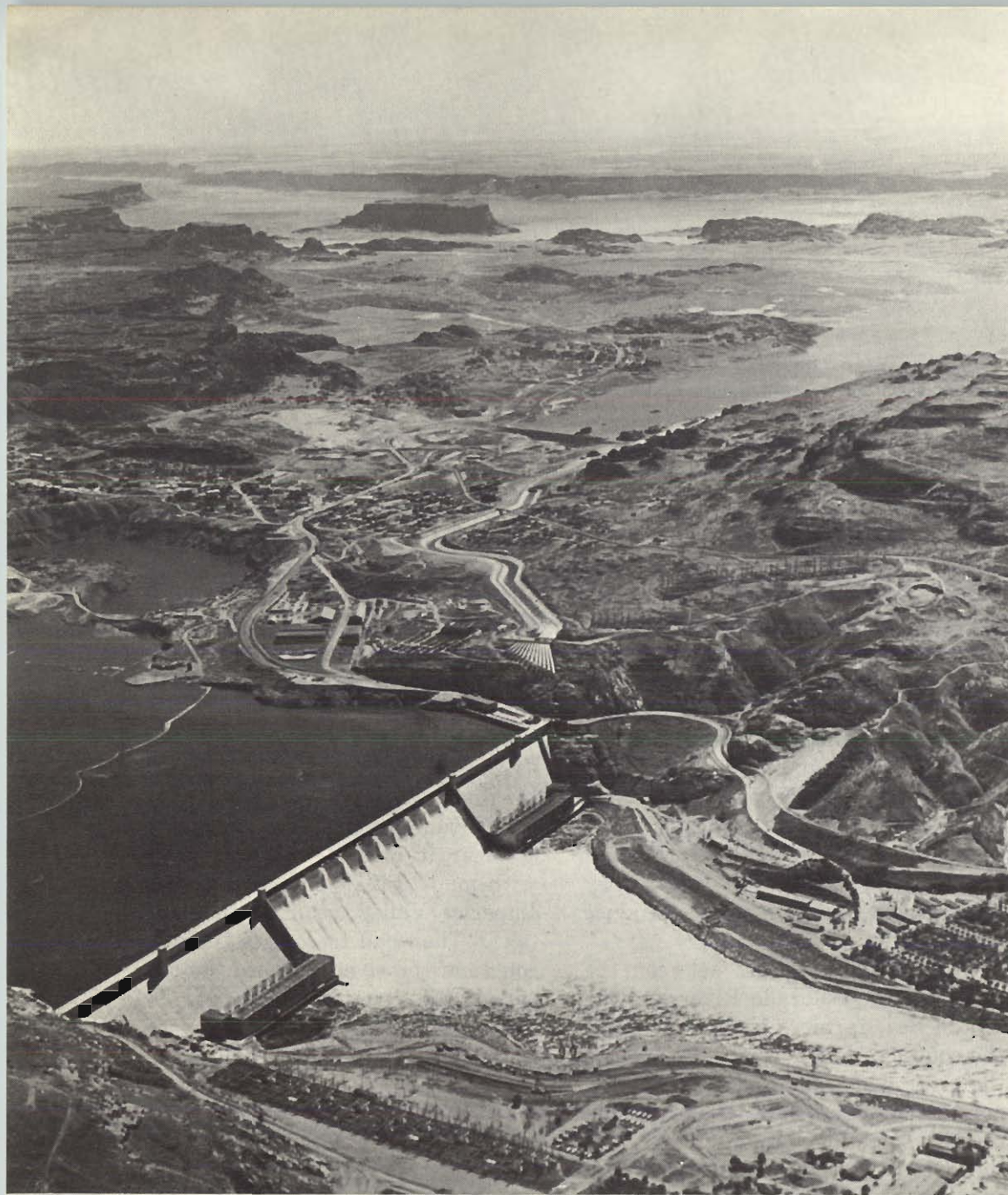
Over 4,000 feet long, Grand Coulee Dam is the largest concrete structure in the Western Hemisphere. It dams the Columbia River, source of the nation's largest reclamation project. Electricity from the dam's power plant is important to the Pacific Northwest, since these states have little coal or oil for fuel.
