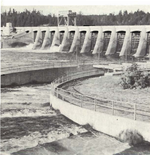
Fish ladders make it possible for salmon to get over Bonneville Dam en route to their spawning grounds.
