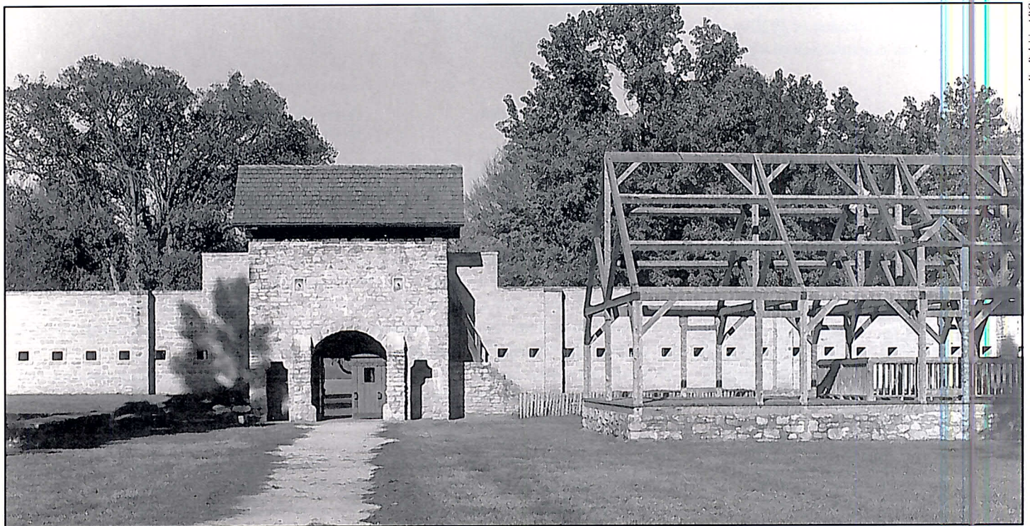
Interior of Fort de Chartres with ghosting of the Government House in right foreground.
