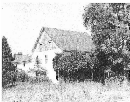
The Davern home is located on the north side of the Davern Road. It was built in 1800 by William Keese, a brother of Richard Keese.
