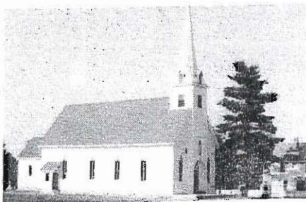
St. Augustine's Church is located on the north side of North Main Street. This lovely building is across from the library.
