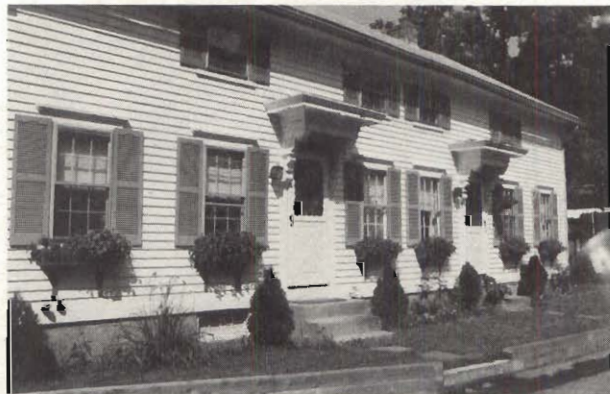
Hope Company Millhouse, Type D (ca. 1885), 10-12 Ives Street. Photograph, June, 1994. One of four 2-story, two-family millhouses, built on a hillside lot acquired by the Hope Company in 1873. Identical entrances have projecting Victorian hoods with heavy curvilinear brackets.
