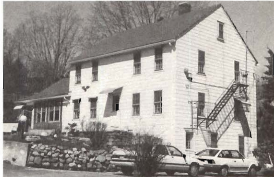
Captain Rufus Hopkins House/Hope Boarding House (ca. 1767 et seq.), 34 Main Street. Photograph, March, 1994. This Colonial house, built for Captain Rufus Hopkins, manager of the Hope Furnace for nearly forty years, became a boarding house for the Lonsdale Company, who acquired the mill estate in 1924. It was modified for apartments after 1944.
