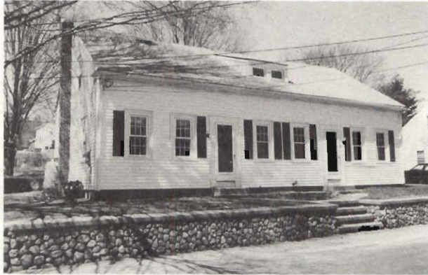
Hope Company Millhouse, Type B (ca. 1821), 33-35 Mill Street. Photograph, May, 1994. A Greek Revival two-family house with paired interior chimneys and a 2-unit shed roof dormer. One of three identical duplexes probably built for Ephraim Talbot, who purchased the mill in 1821.
