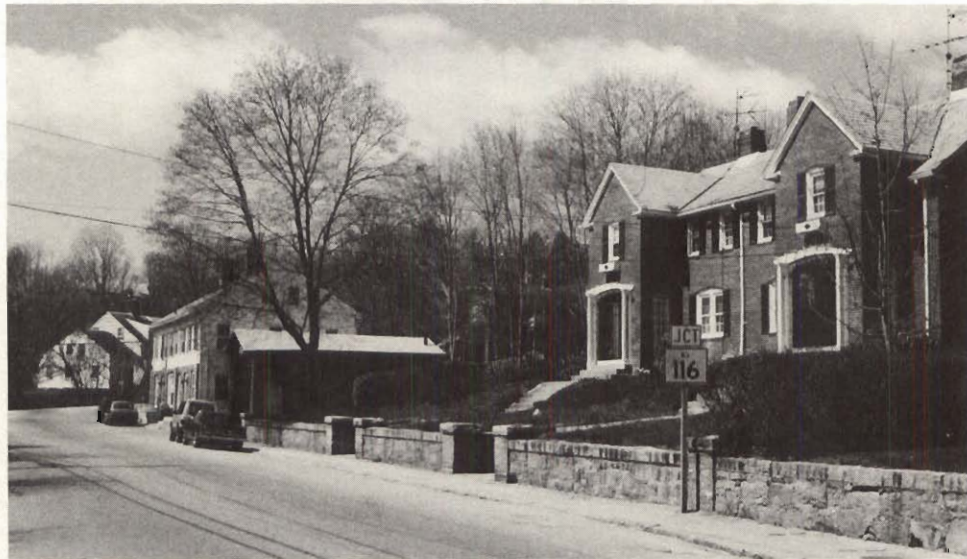
View of Main Street. Photograph, April, 1994. From the far left this view shows the Daniel Fisk House/"Hope House" (ca. 1746 et seq.), oldest house in the village; in the center is the Welcome Matteson Hotel/ Hope Company Store/ United States Post Office (1835 et seq.); to the right is the Overseers' Double House (ca. 1917). Jackson, Robertson and Adams, architects, designed for the Hope Company.
