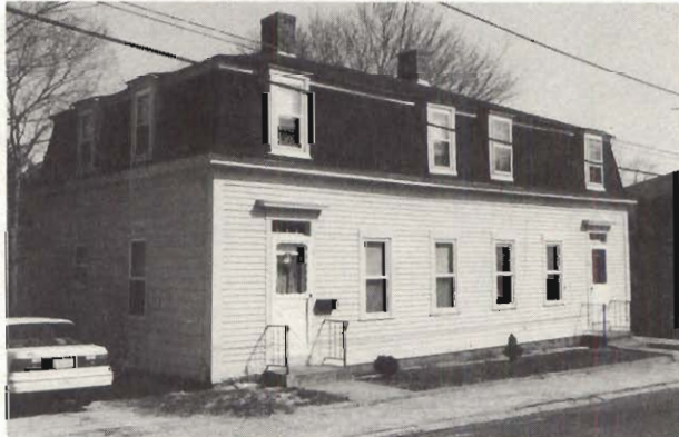
Hope Company Millhouse, Type C (1871-1872), 18-20 Mill Street. Photograph, May, 1994. A Second Empire two-family house with an entrance at each end of the facade. Original door frames and transoms are intact. This is identical to twelve other duplexes built along Mill Street.
