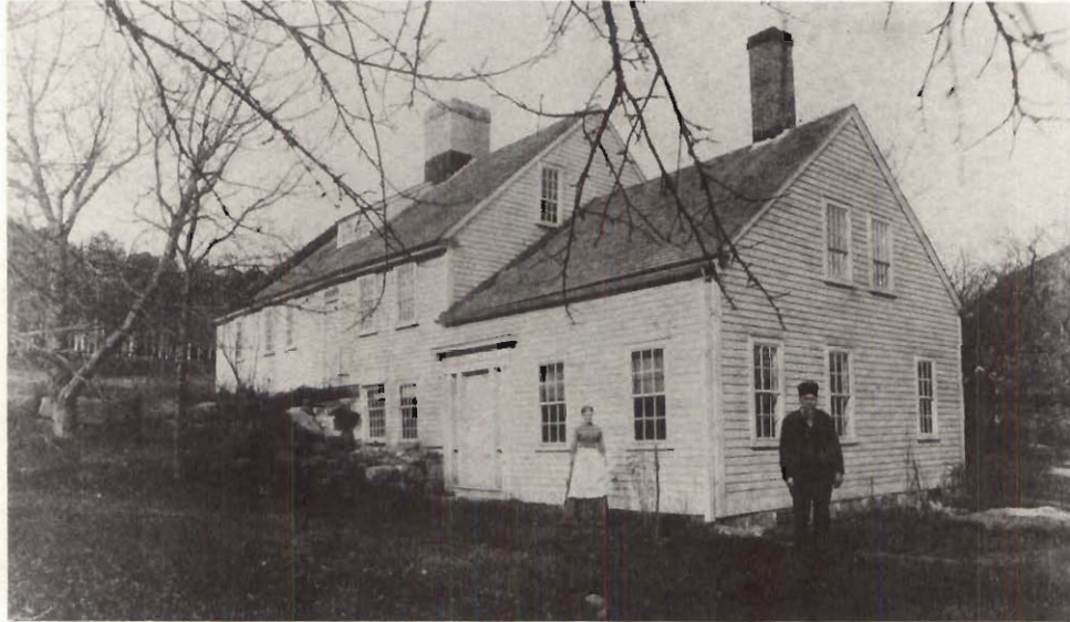
Daniel Fisk House/"Hope House" (ca. 1746 et seq.), 56 Main Street. Photograph ca. 1890, collection Fred Faria. View to the northeast of this Colonial style house. A village landmark, it was built in three sections. On the left is the original south-facing section; on the right is the ell added about 1840; and in 1909 Alice M. Howland, a village benefactor, added a north ell.
