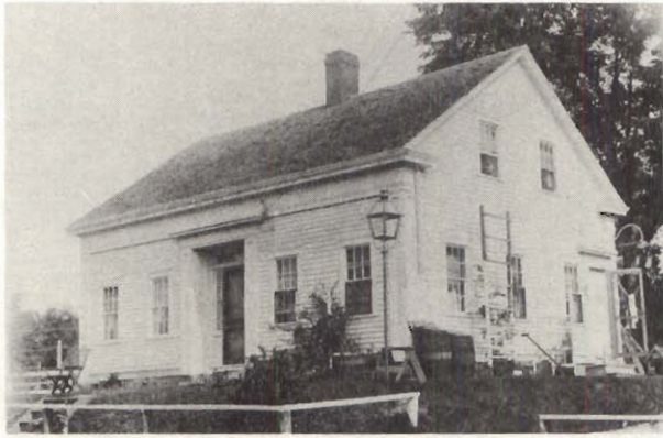
Wilbur-Young House (ca. 1850), 23 High Street. Photograph, ca. 1880, collection Adele Hart. View northwest of the original appearance of this 5-bay, Greek Revival cottage. Typical of eight cottages which were built along High Street for merchants and professionals from the 1840s to the 1860s.
